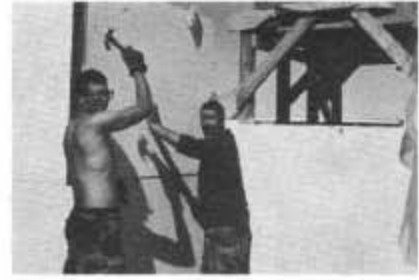
Capt Leser and SGT Bellanger building a shower facility.
