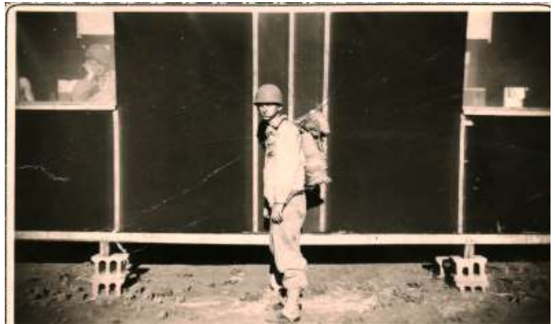
Lewis at Camp Barkeley. To speed construction of training camps, the Army built temporary buildings with wooden frames and tar-paper walls. Hot in the summer, cold in the winter, drafty all year round, they were the bare minimum Lewis Collection, ACHH.
