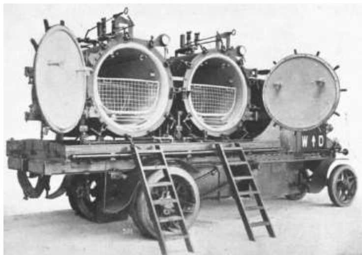
The Foden-Thrush disinfector. Laundry was loaded in the wire baskets, which were steamed to kill lice and their eggs.
