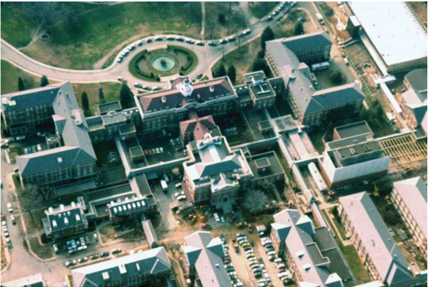
▲ Aerial view of old hospital facing south. The buildings at the bottom of the picture were demolished to make room for the new hospital.
