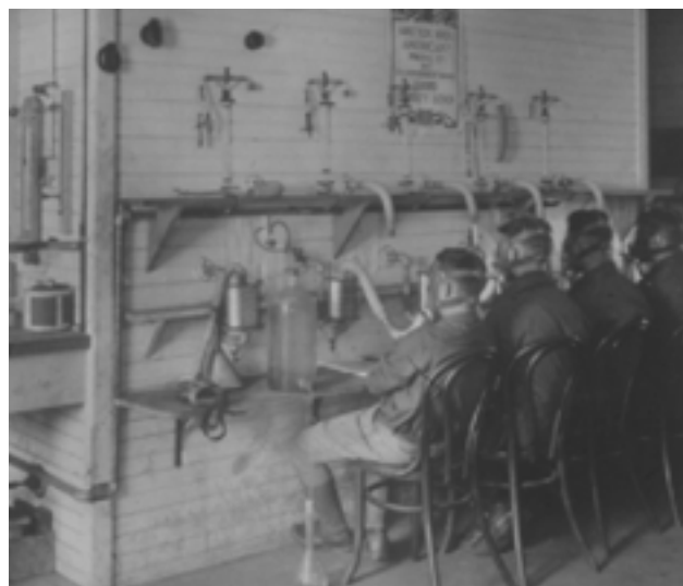
Fig. 3-10. The men are testing experimental canisters, probably performing a primitive form of quality assurance for equipment to protect against chemical warfare agents. Photograph: Courtesy of Chemical and Biological Defense Command Historical Research and Response Team, Aberdeen Proving Ground, Md.
