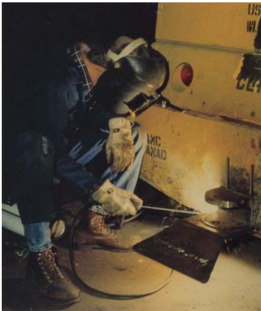
Fig. 12-5. Any process that involves the burning of metallic lead is considered to be a high-risk operation. Steel or stick welding can generate high concentrations of lead fumes and place the worker at risk of lead poisoning. Source: US Army, Anniston Army Depot, Anniston, Ala.
