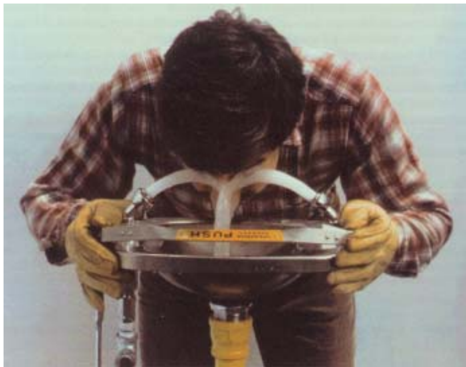
Fig. 8-15. Eyewash fountains and showers should be (a) located within 50 ft of a potential chemical hazard, (b) accessible, and (c) painted high-visibility colors. The hand- or foot-operated valves must allow the eyewash fountain or shower to remain turned on after being activated. Because chemical trauma to the eyes can cause severe spasm of the lid musculature, victims may be unable to open their eyes by themselves. Workers in chemically hazardous areas should be instructed on assisting injured coworkers at eyewash fountains.
