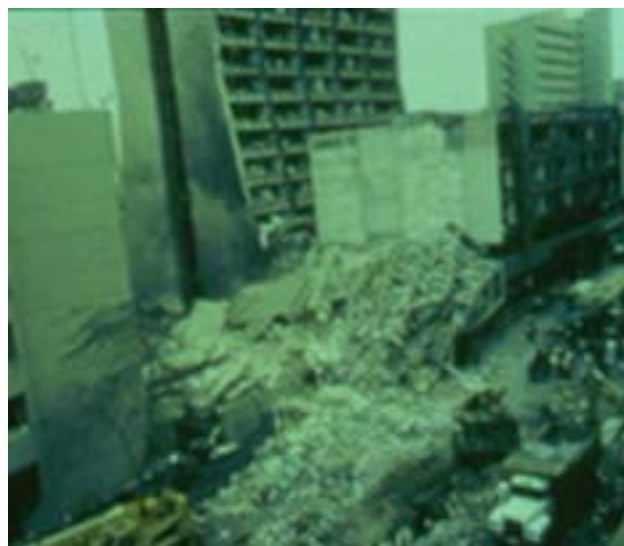
Fig. 24-2. (a) The bank building pictured was adjacent to the US embassy in Kenya before the terrorist bombing on August 7, 1998. (b) After the explosion, the same bank building (rear) has lost of most of the windows on the side closest to the explosion.
