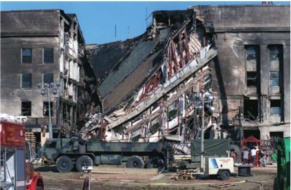
Collapsed wedge on Pentagon’s west side, 11 September 2001. Photograph: Public Affairs, Office of the Surgeon General, US Army.
