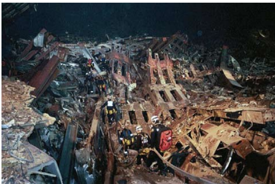
Federal Emergency Management Agency (FEMA) search and rescue team on the rubble pile late at night.
