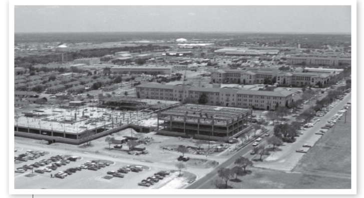
Construction at about 40% complete (U.S. Army Photo, AMEDD Museum Collection)
