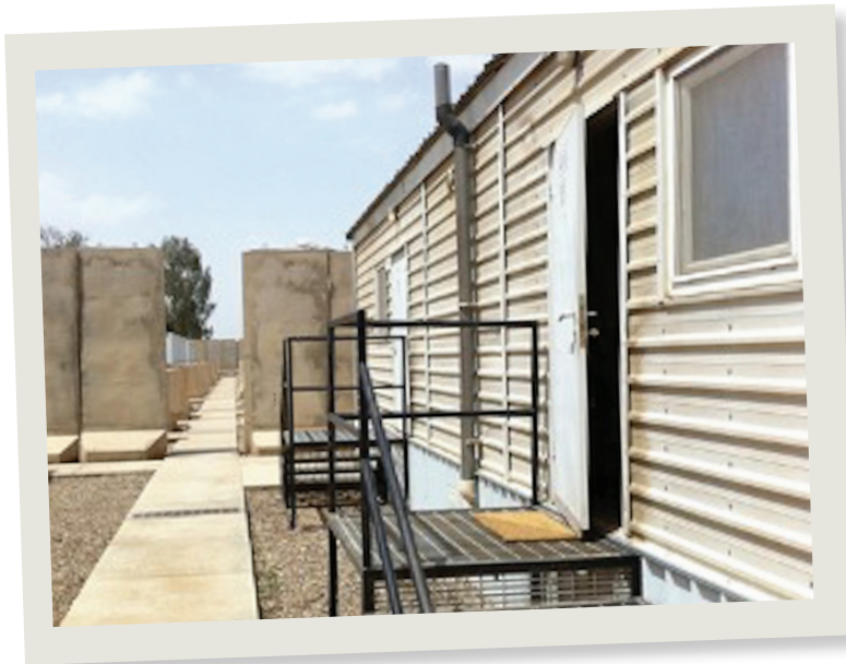
[Figure 5.24] Containerized housing units with sidewalks surrounded by rocks at Sather Air Base in Baghdad, Iraq. Photograph courtesy of Jeff Clemons, MD.
