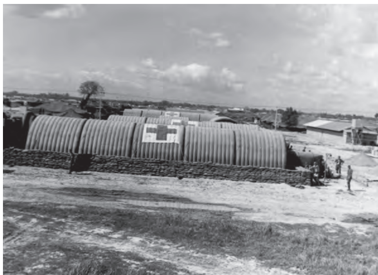
FIGURE 8-2. [Bottom] 45th Surgical Hospital Admission/Disposition Section—a five-section inflatable shelter. Photograph courtesy of the Army Medical Department Center of History and Heritage, Fort Sam Houston, Texas, Image #MU-VN-B1-002.
