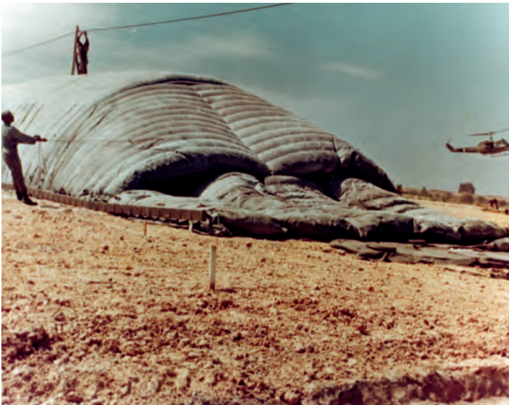
FIGURE 8-3. 45th Surgical Hospital. Inflation of the units using an air supply from the utility pack with connected valve manifold system. Note the UH-1 "Huey" helicopter in the background. Photograph courtesy of the Army Medical Department Center of History and Heritage, Fort Sam Houston, Texas, Image #MU-VN-B1-003.
