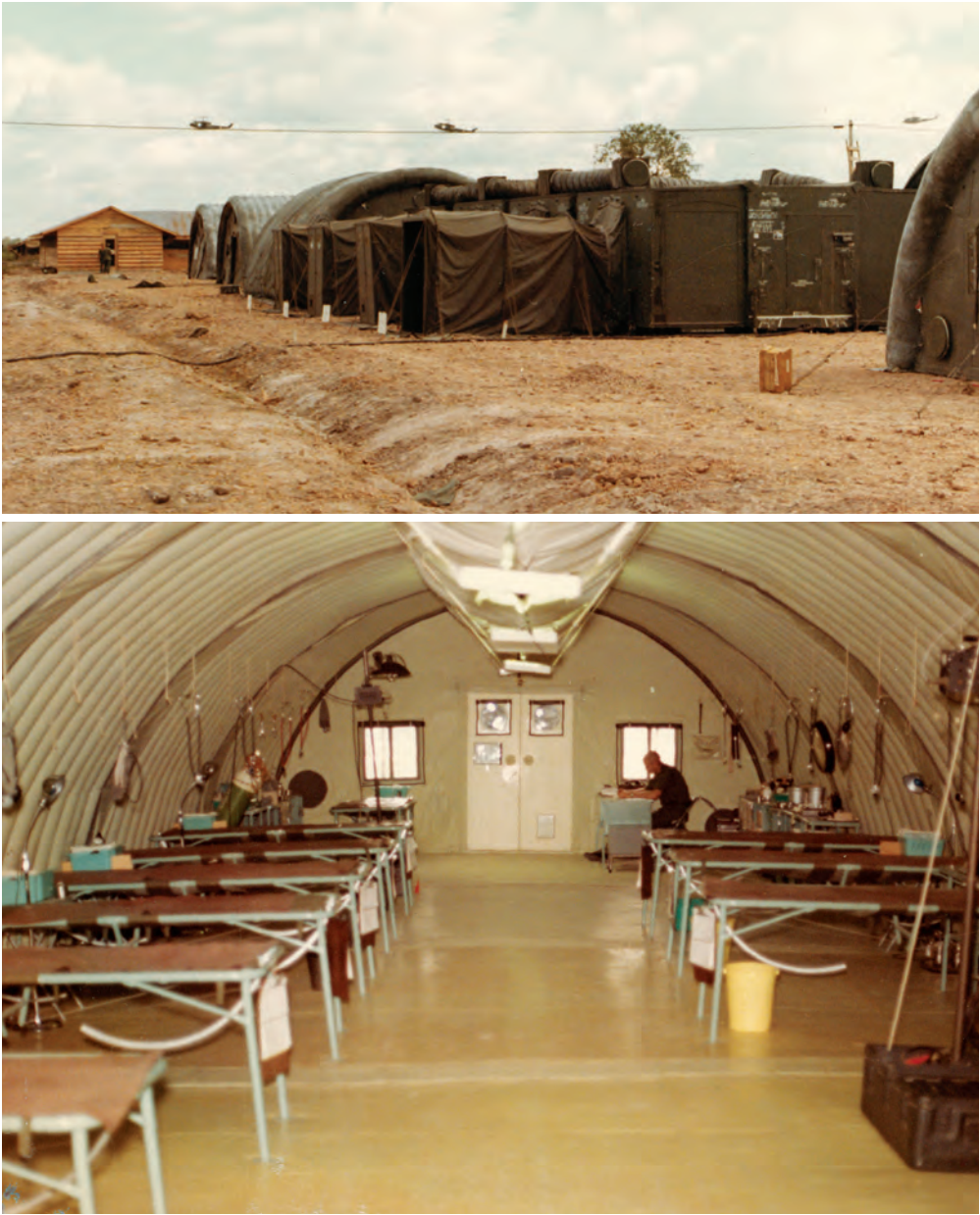
FIGURE 8-6A. [Top] MUST (Medical Unit, Self-Contained, Transportable) surgical complex. Three complete surgeries and a sterile preparation area constitute the four expandable units. Photograph courtesy of the Army Medical Department Center of History and Heritage, Fort Sam Houston, Texas, Image #MU-VN-B1-007.
