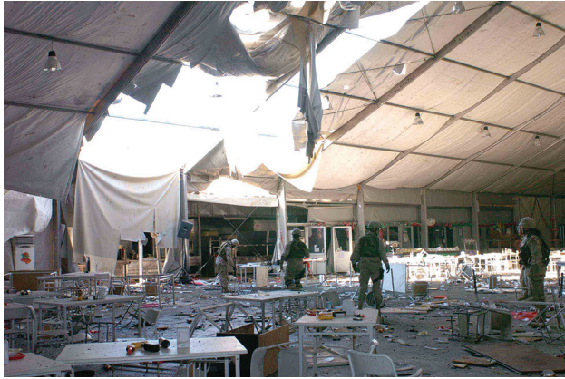
Figure 7-2. Mosul dining hall human-borne improvised explosive device site in December 2004.
