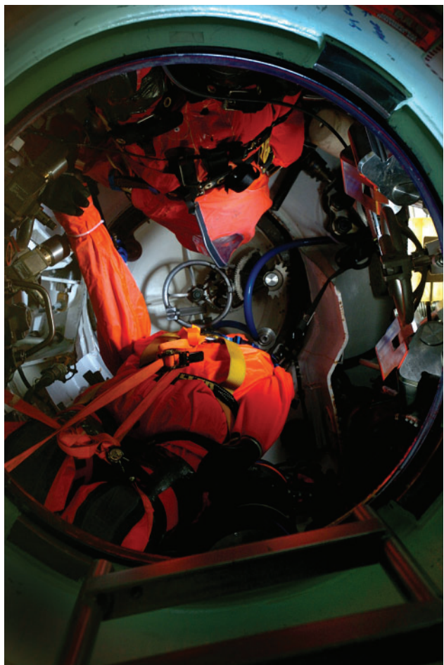
Figure 19-6. Instrument mannequins dressed in MK 10 submarine escape immersion equipment suits inside an engine room logistics escape trunk await the start of General Dynamics' Electric Boat Division fully instrumented trunk test aboard the Virginia-class nuclear powered fast-attack submarine USS Virginia (SSN-774). Reproduced from US Navy news photo 040821-N-2653P-001.
