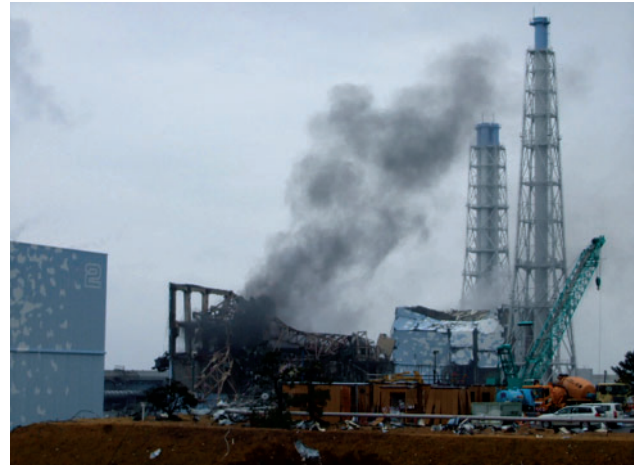
Figure 22-20. Reactor buildings 3 and 4 at Fukushima Daiichi nuclear power station following the fire and explosion that occurred when cooling water was disrupted due to flooding following the earthquake and tsunami. Reproduced with permission from the Tokyo Electric Power Company.
